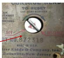
The slot and arrow indicator on the reset component above aligns with the status of the CO<sub>2</sub> bottle.
